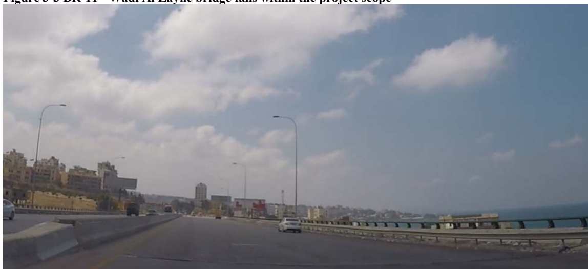
Figure 3-3 BR-11 - Wadi Al Zayne bridge falls within the project scope
