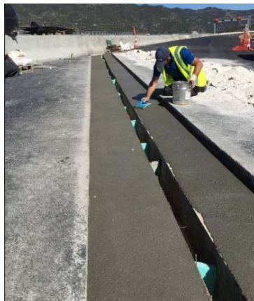
Photo 2 Levelling of surface below the expansion joint
