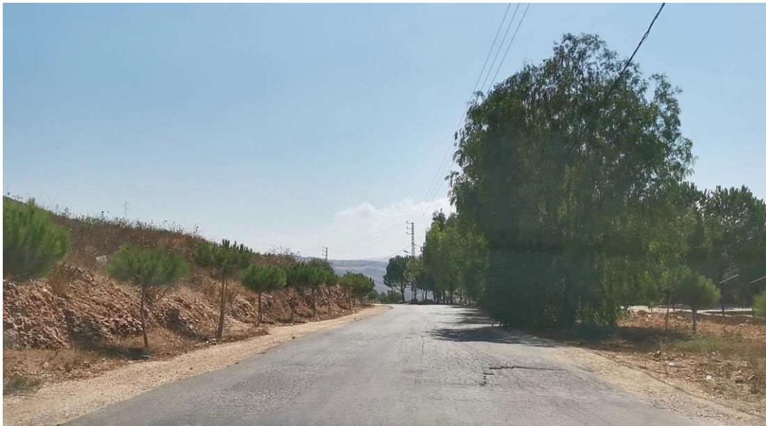
Figure 4-7: Observed trees along the road L3-BW-RD6b (Yohmor- Qellya)
