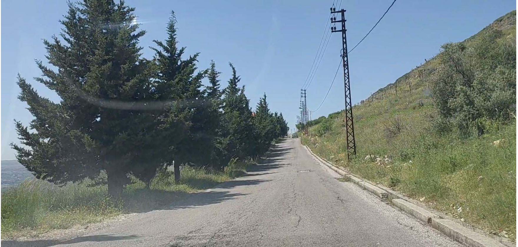
Figure 1: Cypress trees along the Road at Sta. 4+200
