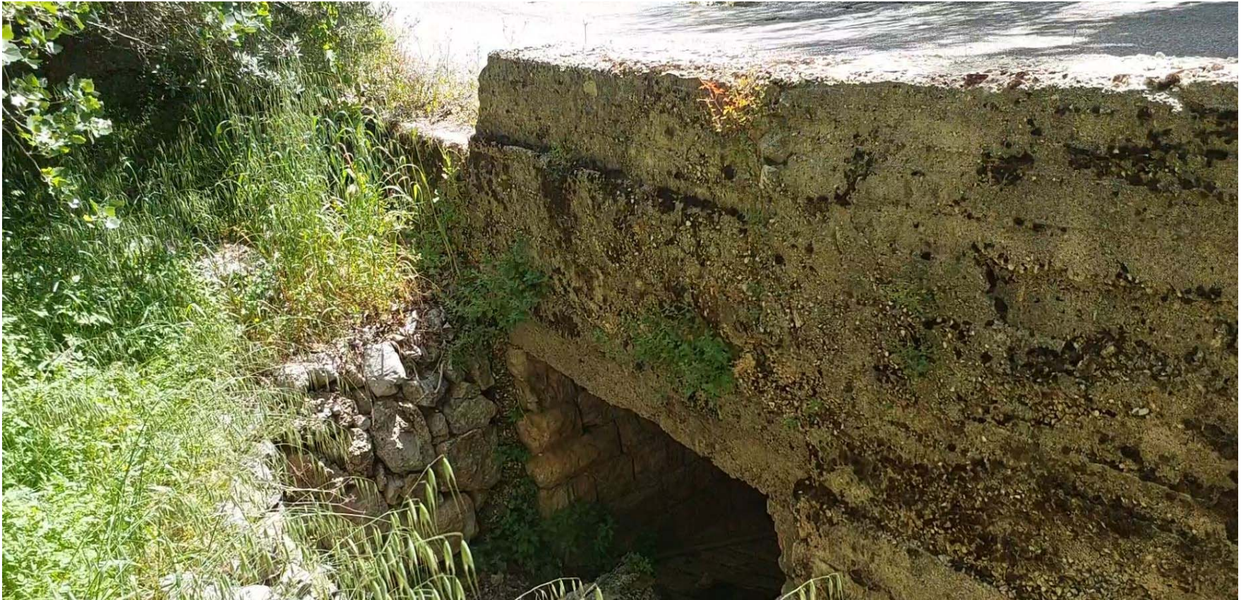
Figure 2: Pipe Culvert at Sta. 3+610
