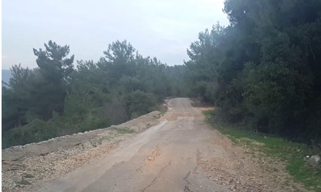
Figure 3-5: Road L3-JE-RD01-a-1, L3-JE-RD01-a-2, L3-JE-RD01-a-3 (Azour-Tiid-Harf-Btedine El Laqch-(To Saida-Jezzine Road)
