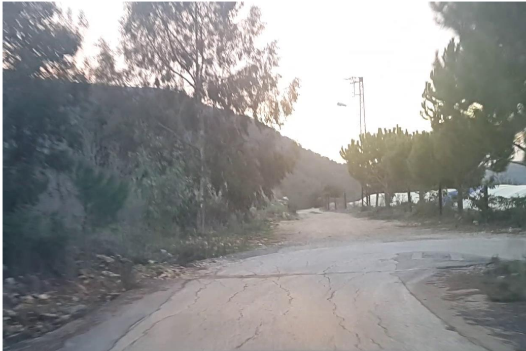
Figure 3-6: Road L3-JE-RD01-a-1, L3-JE-RD01-a-2, L3-JE-RD01-a-3 (Azour-Tiid-Harf-Btedine El Laqch-(To Saida-Jezzine Road)
