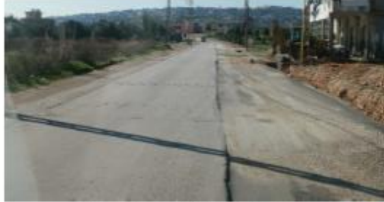
Under construction utility infrastructure
