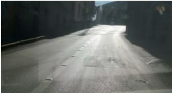
Narrow section, polished asphalt, bad patching and corrugated trench
