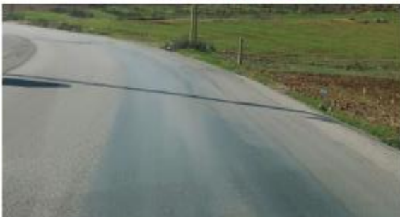
Polished asphalt with bleeding ravelling and bad trench repaving at left and sunken at right
