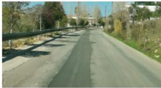
Bleeding, trench in the middle, deformed guardrails at left
