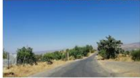
Hasbaya Road 1 – Sta 0+100
