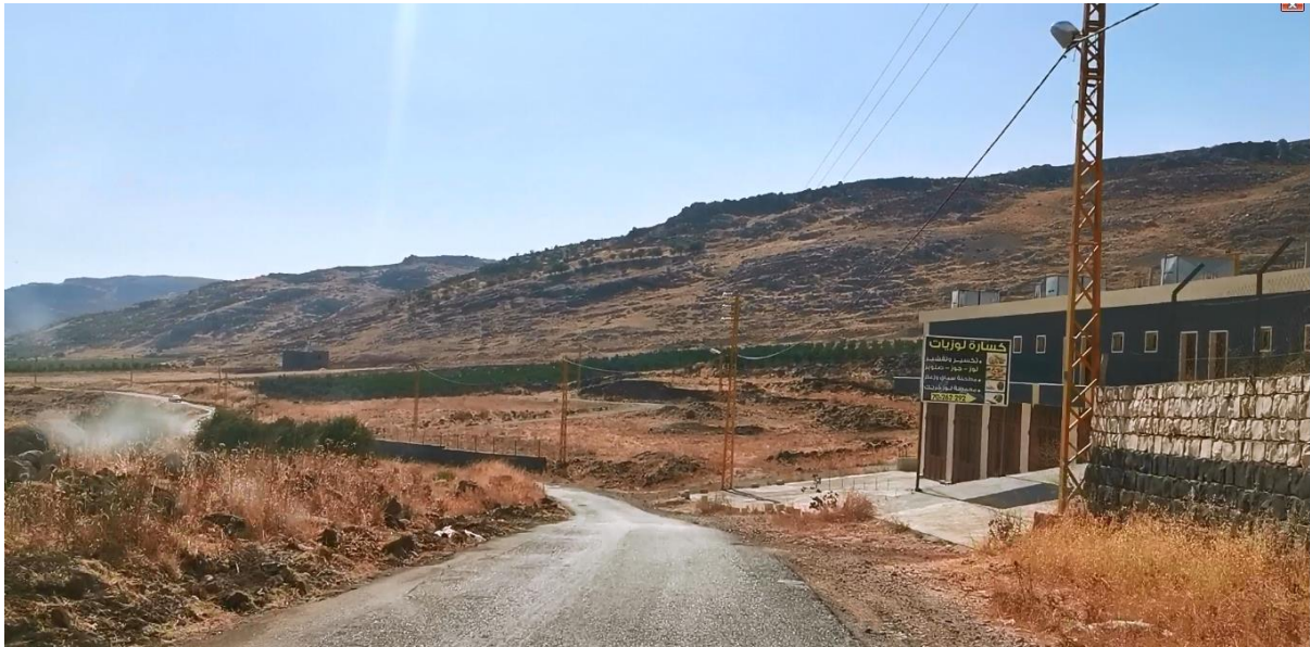
Figure 4-17: Almond Crusher on Road L3-RA-RD04 (Station 3+800)
