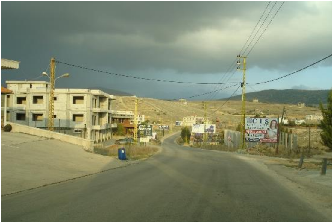
Figure 3-7: Road L3-RA-RD01 (Station 2+500 of Dahr el Ahmar – Kawkaba – to Rachaya Hasbaya Intersection)
