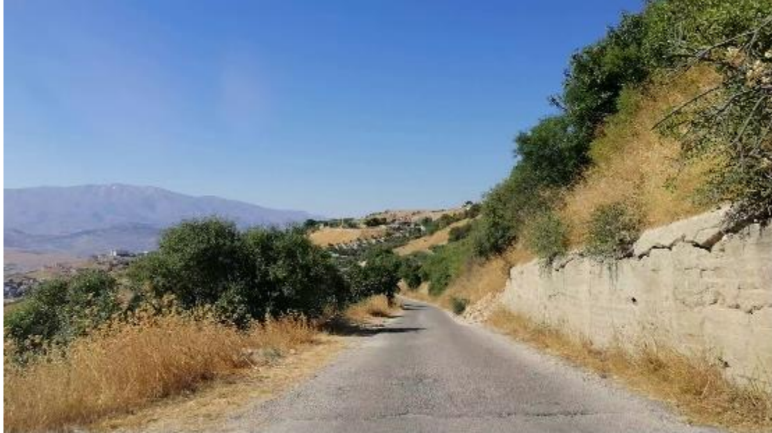
Figure 3-6: Road L3-RA-RD02 (Station 3+150 of Rafid – Bire to Al Masnaa Road)
