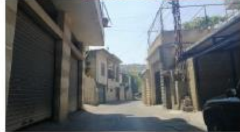
Hasbaya Road 3 – Sta 0+200
