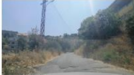
Hasbaya Road 3 – Sta 0+600
