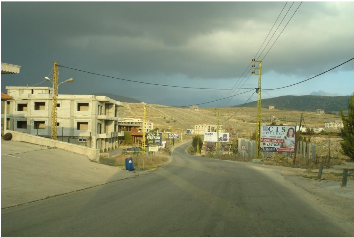
Figure 4-12: Several Shops near Residential Areas on Road L3-RA-RD01 (Station 2+500)
