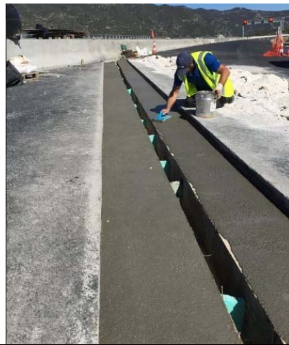
Photo 1 Levelling of surface below the expansion joint
