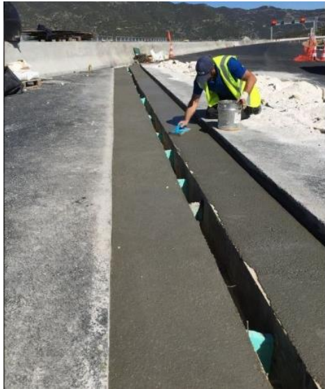
Photo 2 - Levelling of surface below the expansion joint (step 3 above)
