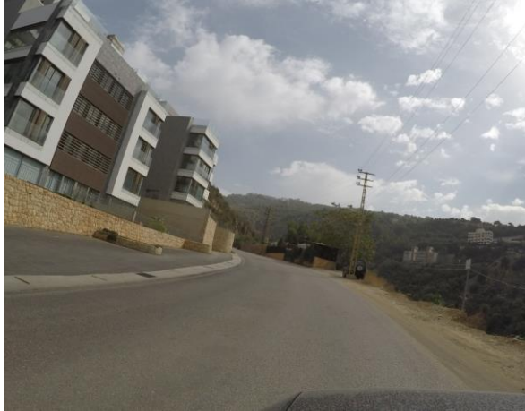
Figure 4-17 Gardens One 282 residential unit
