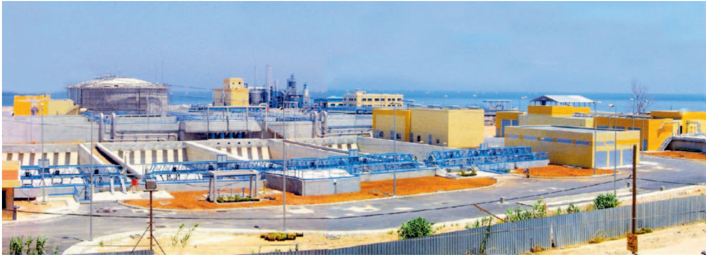
Waste water treatment plant - Tripoli
