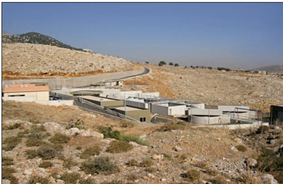
Waste Water treatment Plant - Saghbine
