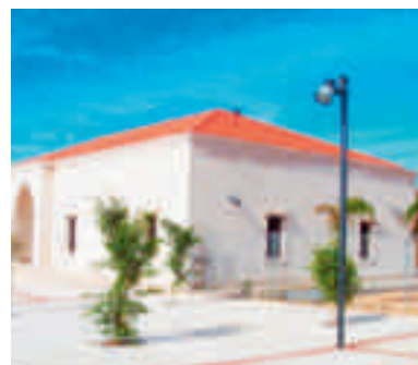
Ansar Municipal Building
