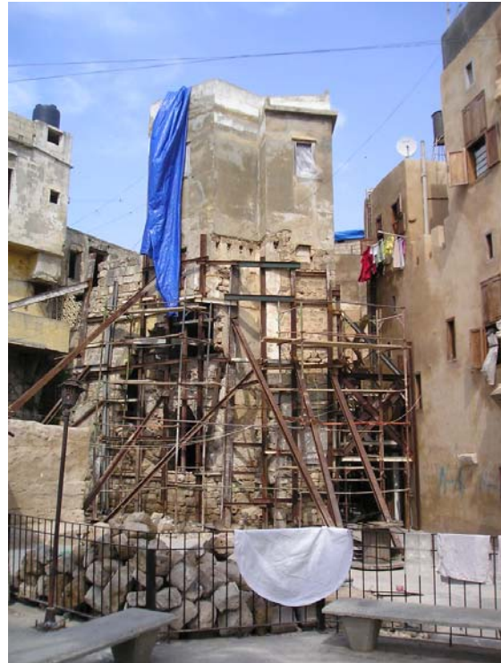
Fig2. Salameh building after consolidation
