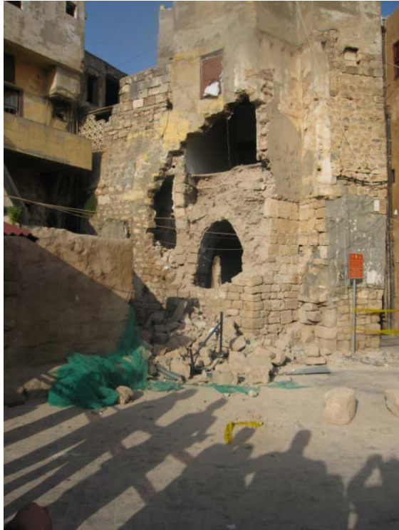
Fig1. Salameh building after the demolition
