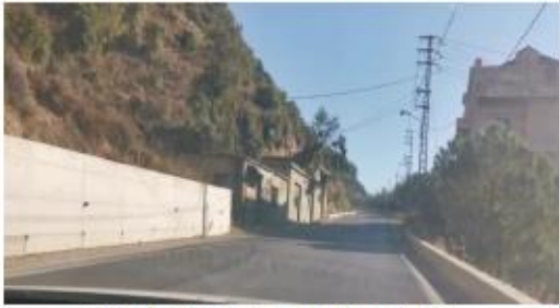
good footwall has been mounted
