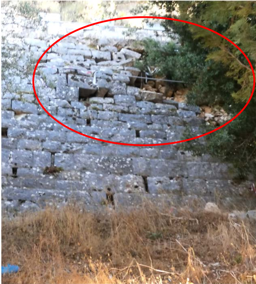
Figure 3-2: Deteriorated stone wall experiencing bulging, wall deterioration and blocks separation
