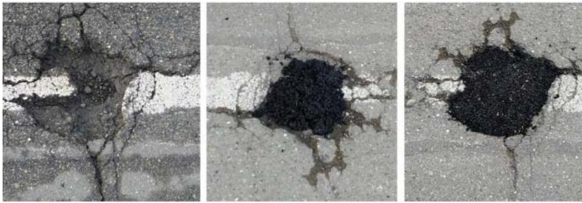
Figure 3-2 Asphaltting shallow potholes
