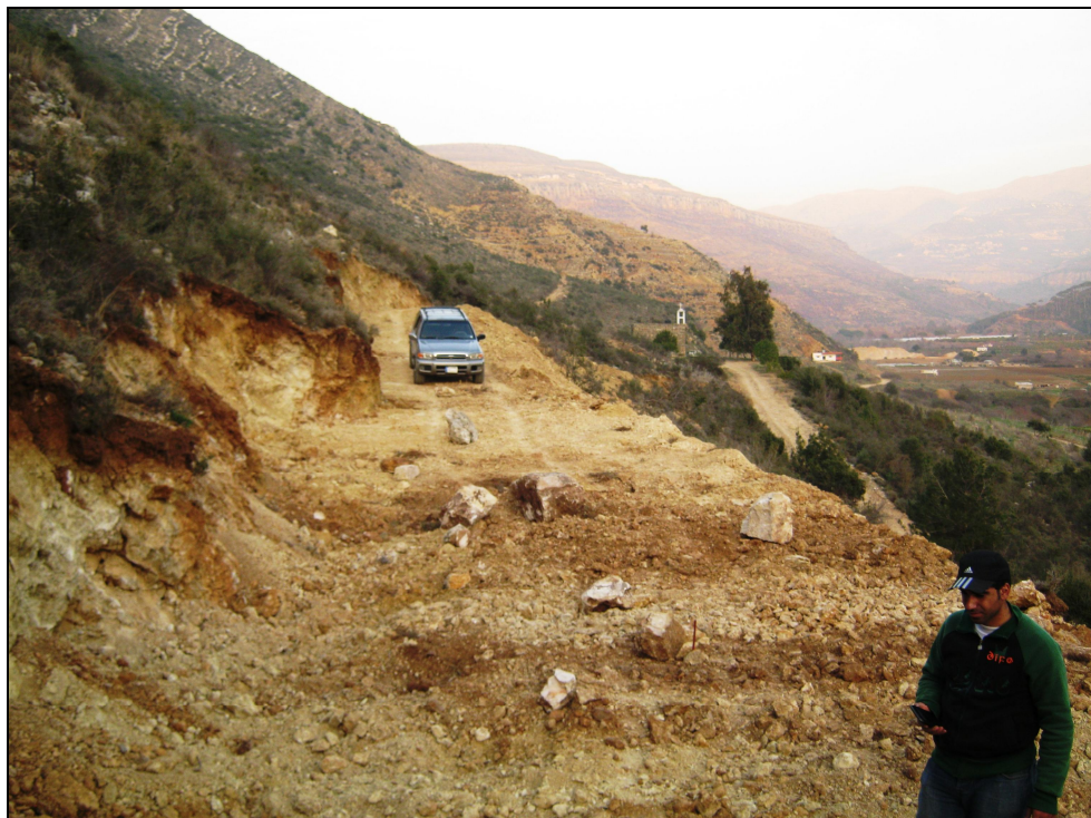
Figure 2: Access rod reaches BHRA1 (right side abutment of the dam)
