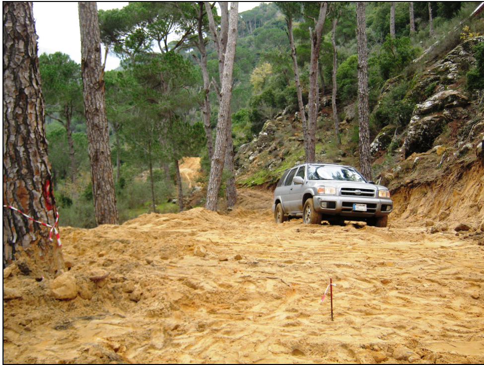
Figure 1: Access rod reaches BHLA2 (left side abutment of the dam)
