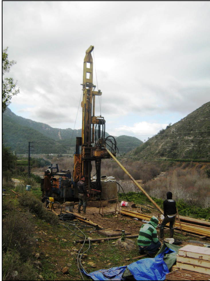
Figure 8: Crawler mounted drill rig used in coring.
