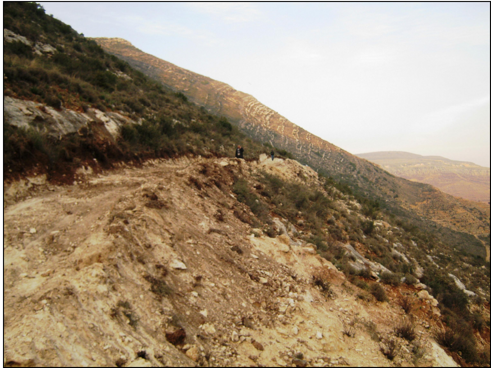
Figure 3: Access road reaches BHRA2 (right side abutment of the dam)
