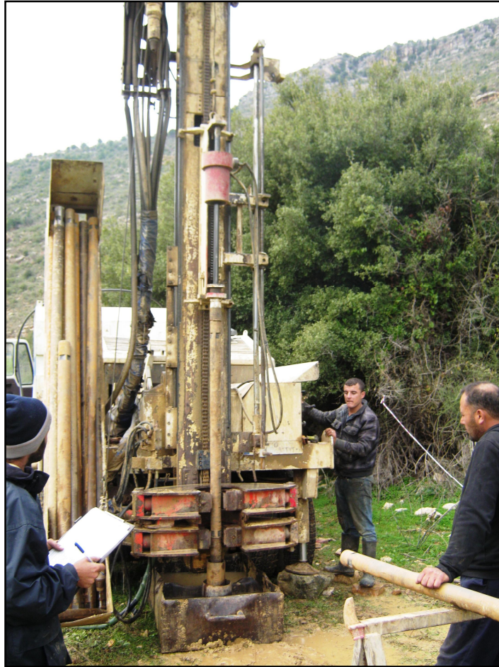
Figure 16: Continuous DCPT probing.
