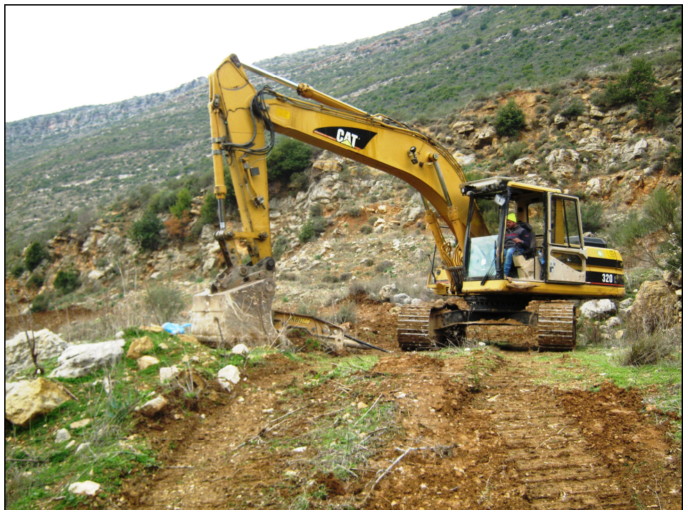
Figure 6: Backhoe excavator equipped with jackhammer
