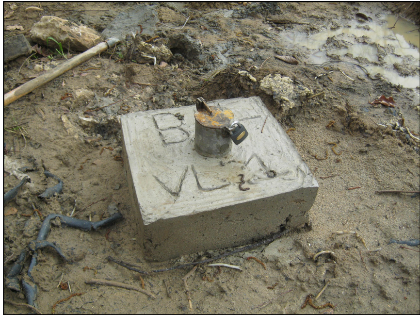
Figure 19: Concrete heading and steel pipe protection
