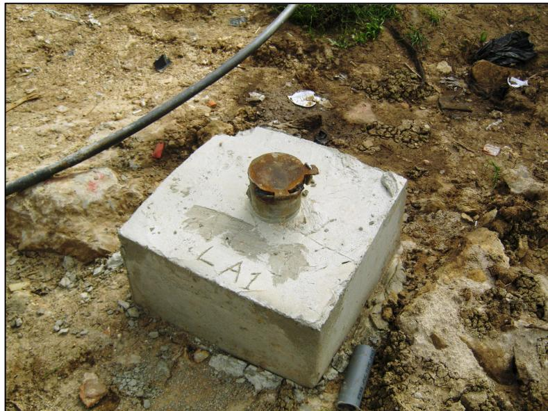
Figure 19: Concrete heading and steel pipe protection
