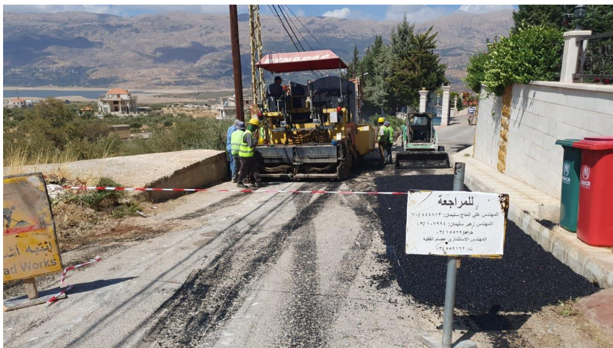
Figure 2: Asphaltting works at line Q2
