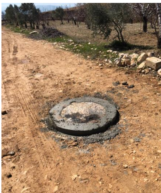
Figure 1: (Left): Raising manhole in Hazerta on agricultural dirt road; (Right): Adjusting manhole cover level to match existing asphalt in Zahle.
