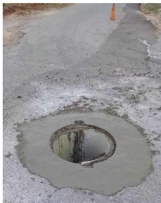
Figure 1: (Left): Raising manhole in Hazerta on agricultural dirt road; (Right): Adjusting manhole cover level to match existing asphalt in Zahle.
