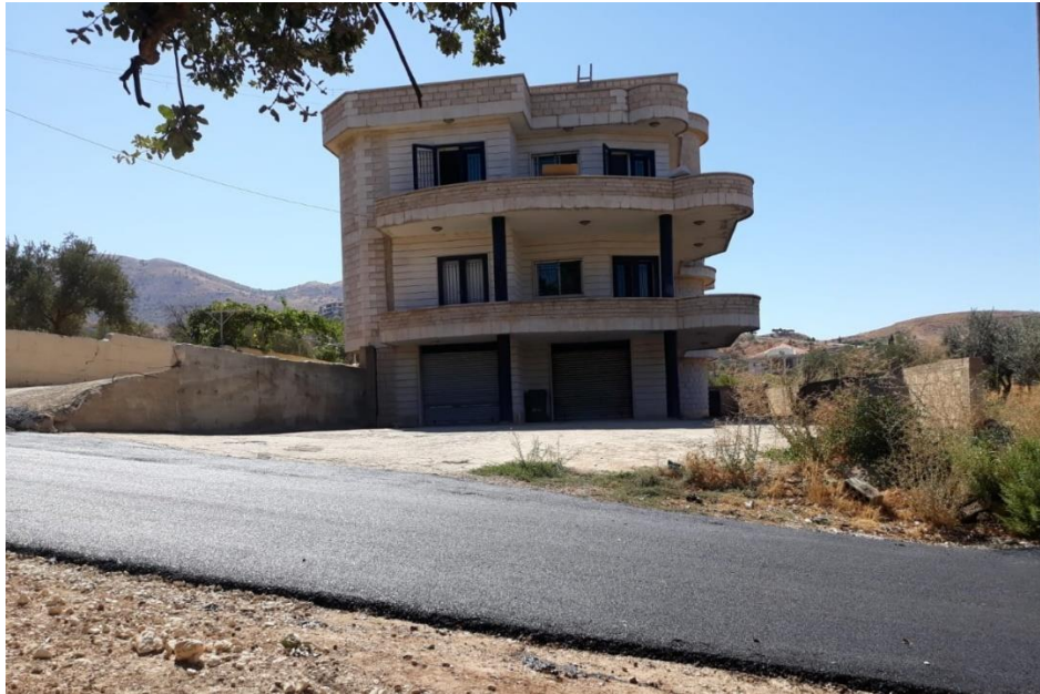
Figure 3: Current road condition facing Ms. Jomaa's house in Baaloul
