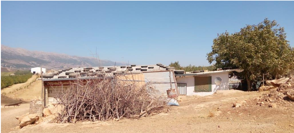
Figure 5: Encroachment on public land at the location of pumping station 3
