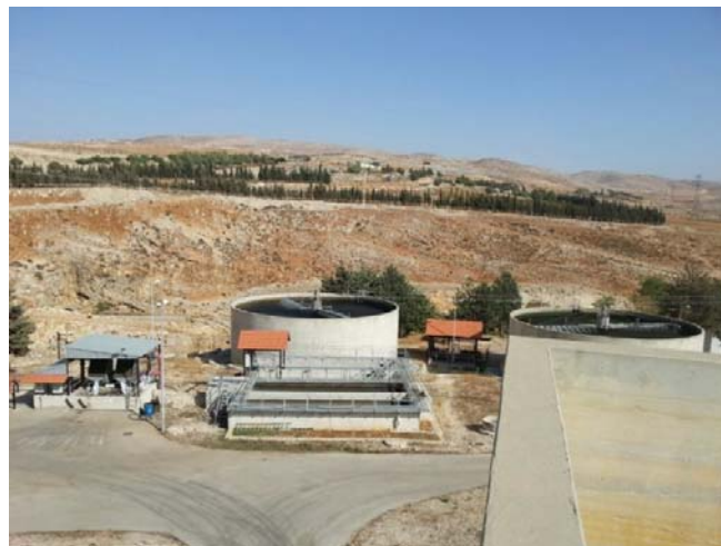
Figure 3-3 Two Trickling Filter Basins
