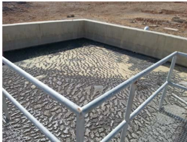
Figure 3-2 Sludge Settling Pond
