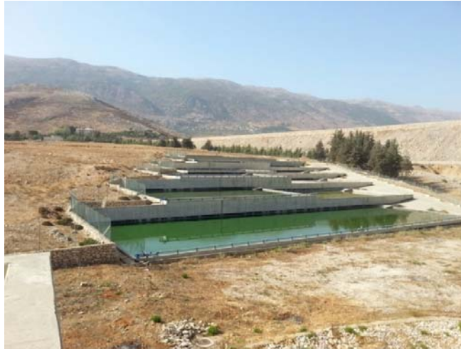
Figure 3-4 Sludge Drying Beds
