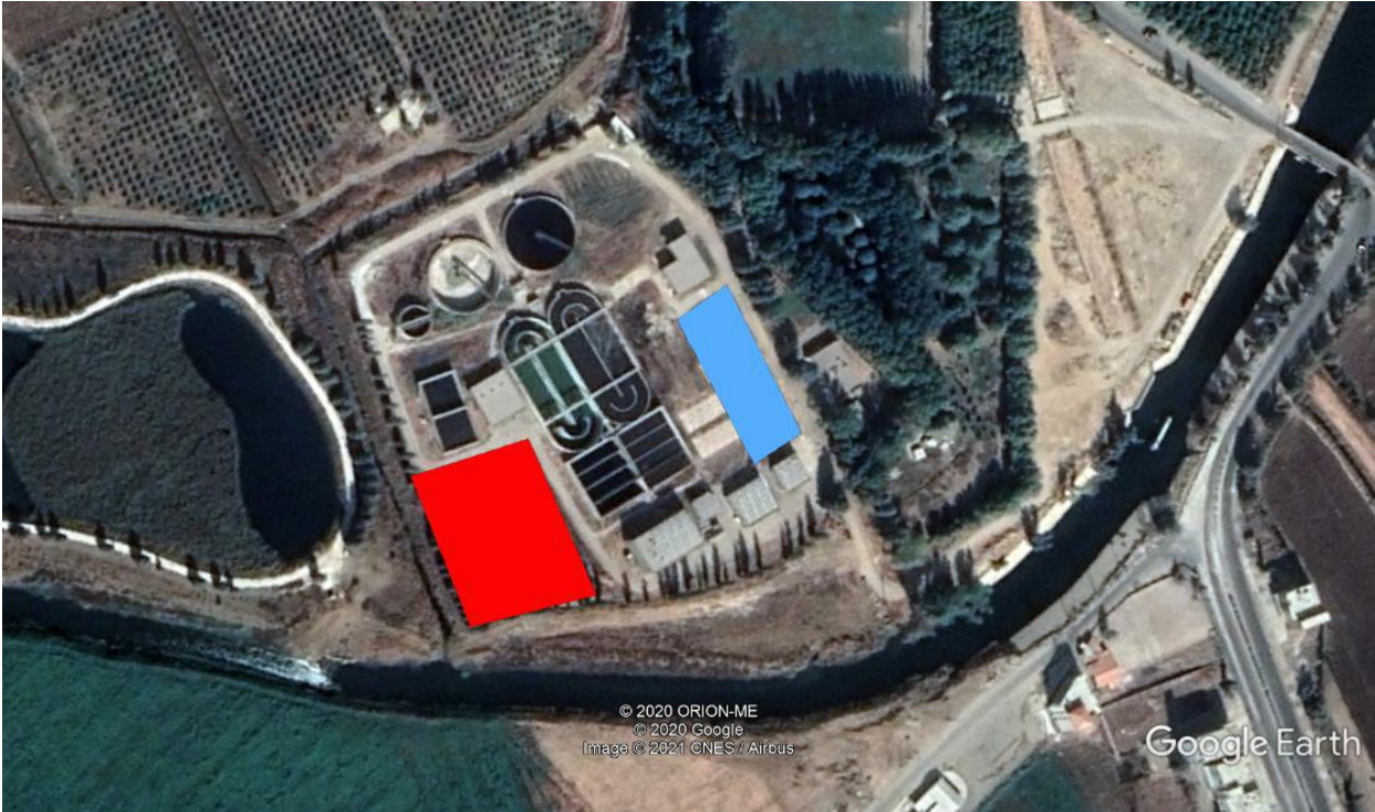
General Layout of the solar drying and storage for scenarios 1, 2 and 4 at Joub Jannine
