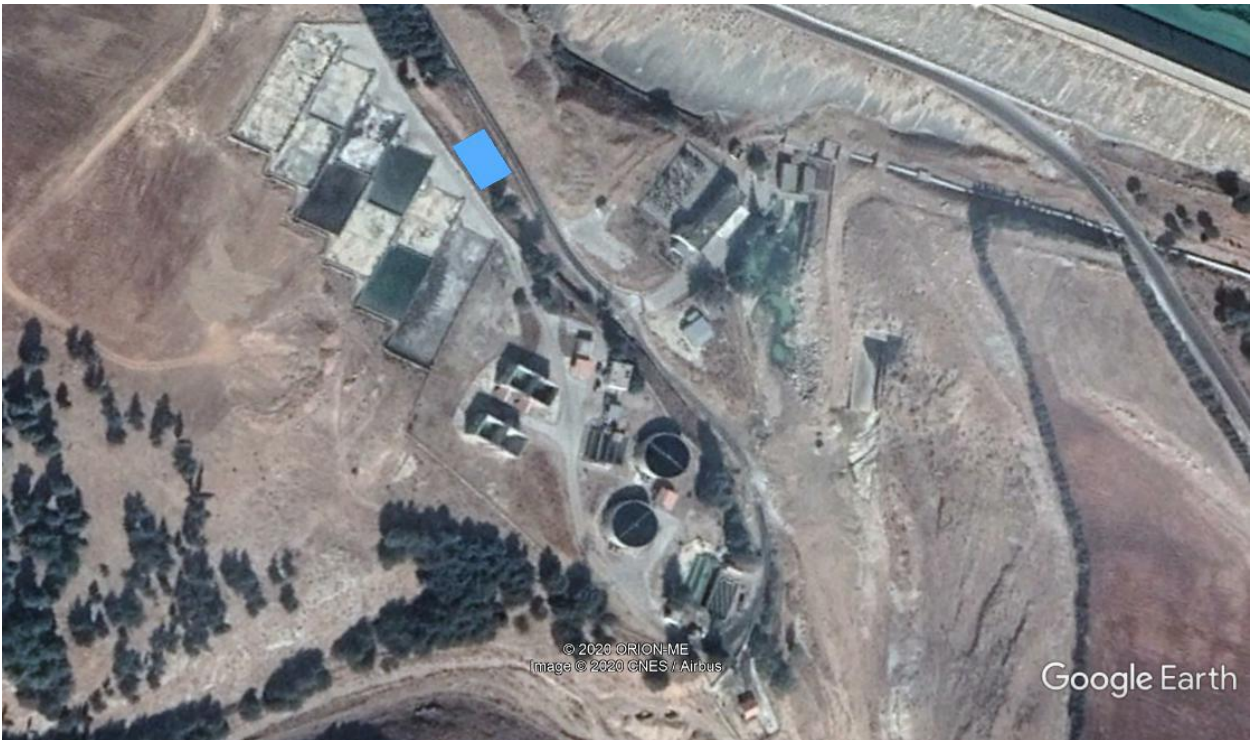
General Layout of the storage (in blue) for scenarios 1, 2 and 4 at Aitanit
