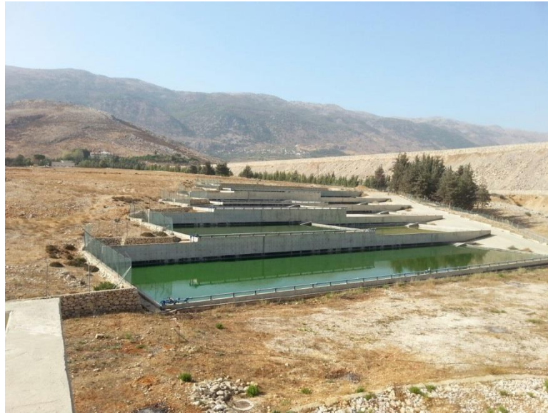
Figure 2-4 Sludge Drying Beds
