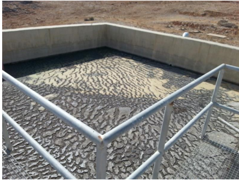
Figure 2-2 Sludge Settling Pond
